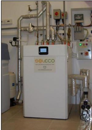
Working from detailed floor plans and SAP reports, H.D. Services Ltd sized the heat pump and designed the water supply borehole and soakaway. The efficiency of both the water supply borehole and soakaway was proved by pumping from one to the other.
