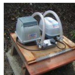
None of our systems employ electrical or mechanical parts within the system itself – all are located outside of the tank, thus avoiding problems associated with wear of electrical or mechanical apparatus in a highly corrosive atmosphere. The treatment process is powered by small air blowers housed in separate 'beehives' or kiosks situated adjacent to the plant and connected to a 230-volt electrical supply from a nearby power source.
